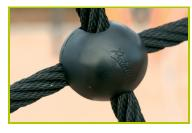
4- The 16mm diameter ropes are made of galvanised steel cable covered with polyester. The cables are linked together and held in place by injected polyamide spheres.
