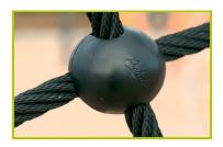
4- The cables are linked together and held in place by injected polyamide spheres.
