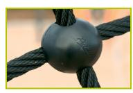
**3- The 16mm diameter ropes** are made of galvanised steel cable covered with polyester. The cables are linked together and held in place by injected polyamide spheres.
