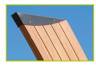
**3-** The shaped beam (95mm thick, 200mm wide and 3.2m high) is made of oven-cured laminated wood with a surface coating; It gives the structure considerable strength.
