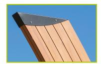
**3- The shaped beam** (95mm thick, 200mm wide and 3.2m high) is made of oven-cured laminated wood with a surface coating; It gives the structure considerable strength.
