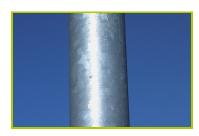
1- The 115mm diameter post is made of galvanised steel.
