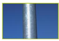
3- The 114mm diameter post is made of galvanised steel.
