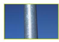
1- The 114mm diameter post is made of galvanised steel.
