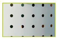
**5- The balcony** is made of 3mm perforated aluminium sheet, coated with polyester epoxy lacquer.
