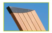
**1- The shaped beam** (95mm thick, 200mm wide and 3.2m high) is made of oven-cured laminated wood with a surface coating; It gives the structure considerable strength.
