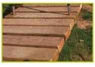
**7- The gangway floor** is made of solid wood planks, with rubber elements between the planks to avoid all risk of catching a finger.
