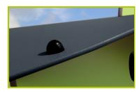
3- The roof is made of 10mm thick polyethylene plates.
