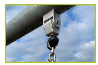
3- The swing bearings are made of stainless steel.
