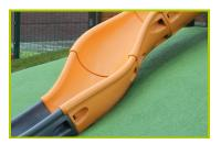
5- The Kayak slide is made of rotomoulded polyethylene.
