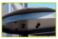
5- The platforms are made from a 12.5mm thick, textured, non-slip compact material
