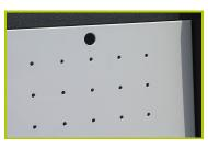
2- The structure is made of painted perforated aluminium liner (RAL 7004), thickness 3mm with 5mm rounds.
