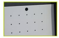
**2- The structure** is made of painted perforated aluminium liner (RAL 7004), thickness 3mm with 5mm rounds.
