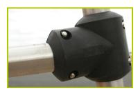
5- Injection moulded polyamide fixings connect the posts with the platforms and the various play features. They are non-toxic, flameproof and U.V. resistant. The thickness of the polyamide makes the equipment both strong and vandal resistant.
