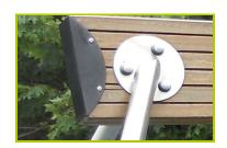
1- The horizontal beam is made of oven-cured laminated wood with a surface coating.
