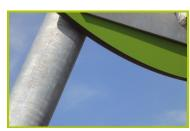
**2- The support legs** are made from 60mm galvanised steel.
