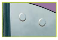
5- Stainless steel version: the play walls bring together a coloured panel and a stainless steel sheet, 1.5mm thick with a patterned surface on both sides to make it scratch-proof. The roofs are made of polyethylene 10mm thick.
