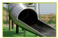
6- The tubular slide is made of stainless steel.
