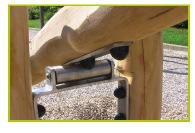
**4- The rocking mechanism** is made of stainless steel.
