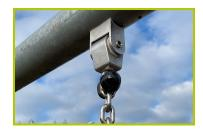
**3- The swing bearings** are made of stainless steel.
