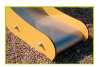
6- The sliding surfaces are made of 2mm thick stainless steel, which is shaped, bent and rolled from one piece.
