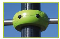
**2- Injection moulded polyamide fixings** connect the posts with the platforms and the various play feautures.
