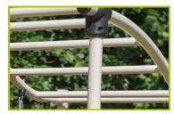
**2- The tubes** are made of epoxy polyester lacquered aluminium (40x40, Ø 30 and Ø 40mm).
