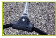
4- The net fittings are made of polyamide. The fittings are composed of two distinct parts for ease of maintenance of individual strands.
