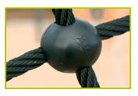
**7- The 16mm diameter ropes** are made of galvanised steel cable covered with polyester. The cables are linked together and held in place by injected polyamide spheres.
