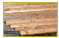
3- The roofs are made from larch logs (80 x 40 mm).
