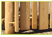
**4-** The panels, the climbing wall, the steps and the tunnel are made from larch (plank sizes 140 x 27mm / 45 x 68mm). Larch is naturally resistant and long lasting.
