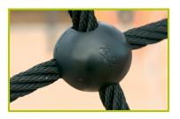
**7- The 16mm diameter ropes** are made of galvanised steel cable covered with polyester. The cables are linked together and held in place by injected polyamide spheres.
