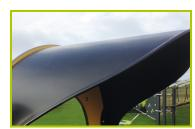
3- The roof (2) is made of aluminium painted sheet.
