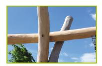
**1- The posts and the horizontal beam** (diameter 120 to 140mm), are made from sap free robinia.
