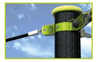
7- Injected aluminium elements are fixed on the posts with self-drilling screws to provide links between the ropes and the posts.
