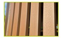
**4- The slatted fences** are made of composite wood (slats of 70 x 30 mm), which is a chip and split resistant waterproof material with UV protection.
