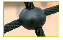
**5- The 16mm diameter ropes** are made of galvanised steel cable covered with polyester. The cables are linked together and held in place by injected polyamide spheres.
