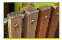
**4- The panels** are made from larch (plank sizes 140 x 27mm / 45 x 68mm). Larch is naturally resistant and long lasting.
