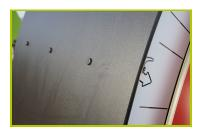
**4- The roof** is made of polyethylene plates 10mm thick.
