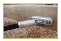
5- The fixings for the nets and chains are made from aluminium.
