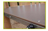
2- The platforms are made from a 12.5mm thick, textured, non-slip compact material (HPL). Further reinforcement is provided by galvanised steel supports, located on the underside of the platforms.
