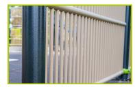
**2- The mesh fencing** is made of painted aluminum. The goal area mesh fencing is made of painted galvanised steel.
