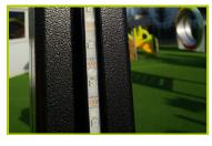
5- The led strip lighting is embedded in a painted steel profile.
