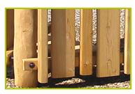
**3- The panels and the steps** are made from larch (plank sizes 140 x 27mm / 45 x 68mm). Larch is naturally resistant and long lasting.
