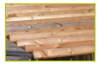
4- The roofs are made from larch logs (80 x 40 mm).
