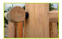
1- The different posts (average diameter: 60 to 80mm / 100 to 120mm / 120 to 140mm) are made from sap free robinia. The robinia is sanded and has had its bark removed. Robinia is naturally rot proof and does not require any additional chemical protection; it is equally extremely resistant to attacks from external sources (insects, fungi, climatic variations), guaranteeing the long term durability of the playground equipment.
