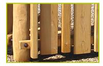
2- The panels, the climbing walls and the tunnel are made from larch (plank sizes 140 x 27mm / 45 x 68mm). Larch is naturally resistant and long lasting.
