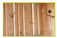
2- The panels, the climbing wall, the gangway, the shelf and the tunnel are made from larch (plank sizes 140 x 27mm / 45 x 68mm). Larch is naturally resistant and long lasting.
