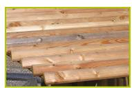
**3- The roofs** are made from larch logs (80 x 40 mm).
