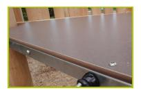
**4- The platforms** are made from a 12.5mm thick, textured, non-slip compact material (HPL). Further reinforcement is provided by galvanised steel supports, located on the underside of the platforms.
