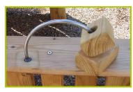
The abacus pieces are made of robinia. The rail is made from 10mm diameter stainless steel.
