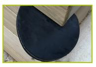
**7- The ears** are made from rubber, 14mm thick.
