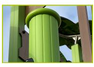
2- The 125mm diameter posts are made of painted galvanised steel. The caps are made of injection moulded polyamide.
