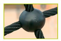
6- The 16mm diameter ropes are made of galvanised steel cable covered with polyester. The cables are linked together and held in place by injected polyamide spheres.
