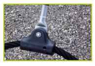
7- The net fittings are made of polyamide. The fittings are composed of two distinct parts for ease of maintenance of individual strands.
