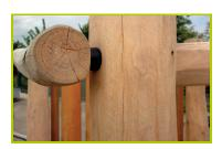
1- The 120/140mm diameter seat is made from sap free robinia. The robinia is sanded and has had its bark removed. Robinia is naturally rot proof and does not require any additional chemical protection; it is equally extremely resistant to attacks from external sources (insects, fungi, climatic variations), guaranteeing the long term durability of the playground equipment.
