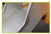
6- The slide is made of stainless steel.
