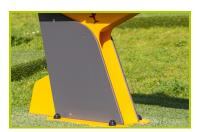
**9- The structure of the equipment** is made of painted galvanised steel. The coloured panels are made from a 13mm thick compact material (HPL). Robust in construction, it has excellent weather and vandal resistance properties.
